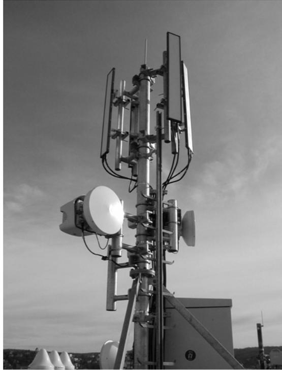
**Figure 13-4: A Base Station Sector Antenna Array**
