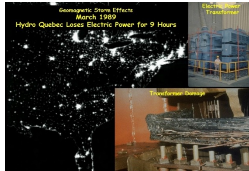
Ground system damage on 13 March 1989
