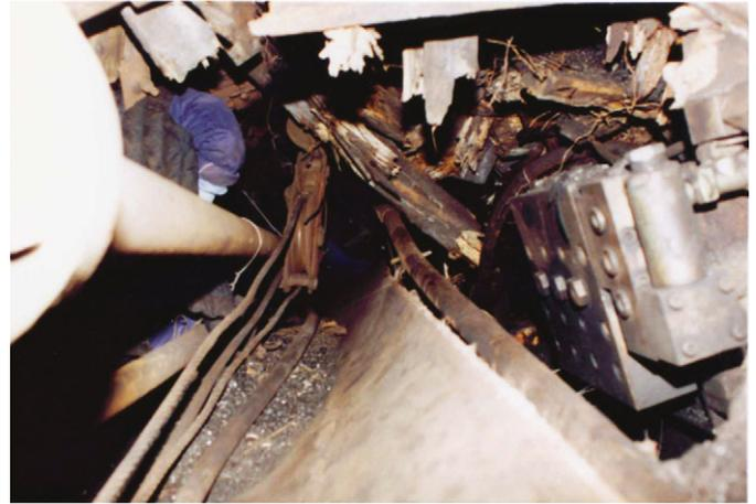
Fig. 13. Damaged drift at 55,001 mining area at Laohutai coalmine.
