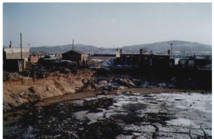
Fig. 14. Sudden roof failure leading the ground subsidence at Laohutai coalmine.
