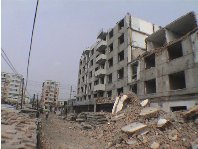
Fig. 15. Demolition of the apartment buildings damaged by rockbursts in Fushun City, Liaoning Province.
